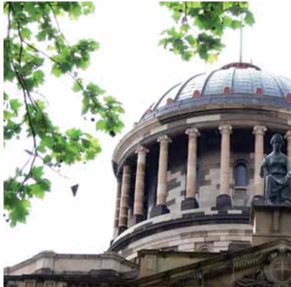
The Supreme Court of Victoria, William Street building.
